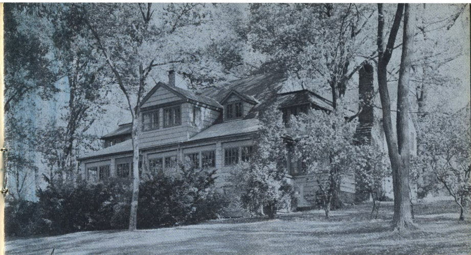
The Main Lodge facing the lake well back from the beach.
