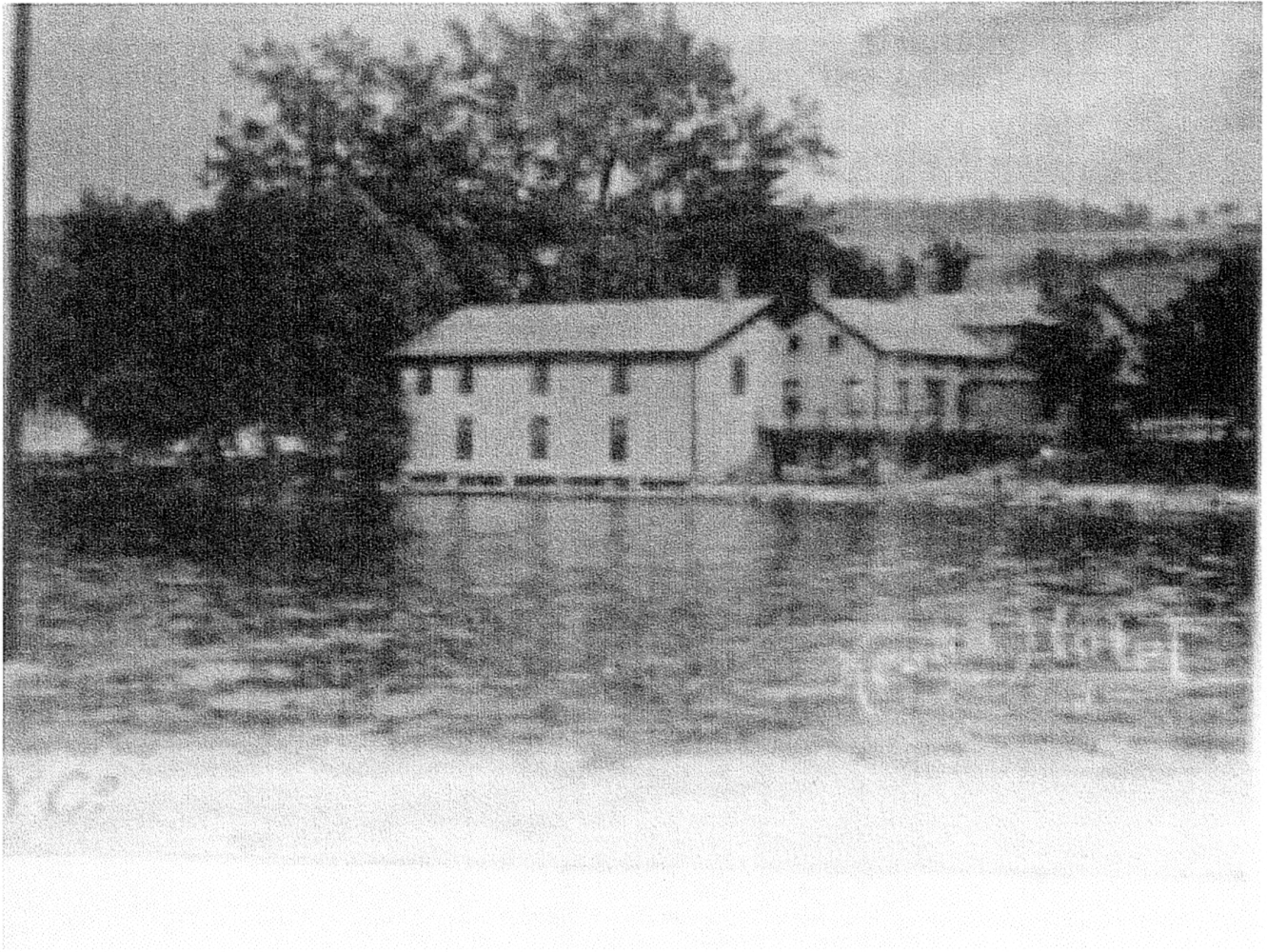
Figure 2. Photo of the "Keuka House" shows what looks like two buildings in the center of the photo. The building at the left was apparently the "Keuka House" and was eventually moved towards the south, remodeled and became the Switzerland Inn, a popular restaurant and establishment for over 100 years. At that time, the "House" was apparently a fishing "resort" and was "kept by Washburn & Wright", according to Anonymous (c.1895). The second building was apparently moved to the north and used as a cottage. The lot remaining was used to construct the Keuka Hotel. Photo from the book "Lake Keuka", Anonymous (c. 1895). Photo courtesy of the Hammondsport, NY Library.
