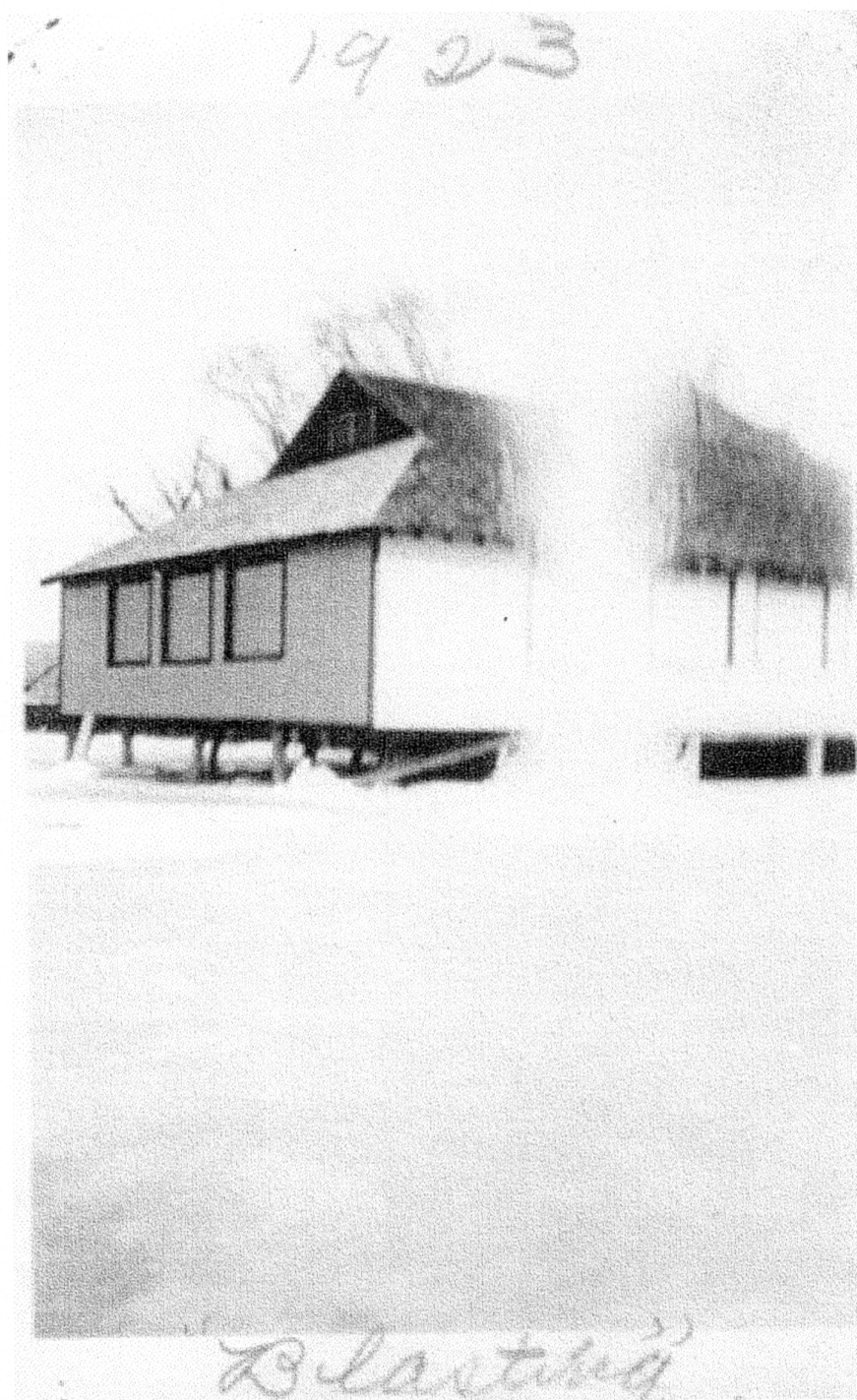
Figure 9. Photograph from 1923 showing ice surrounding the Keuka Dance Hall. Also, note the white vertical gusher in the center of the photo. This was the result of using dynamite to break up the ice which would in turn relieve pressure on the piers. Ice, if not broken up, would pressure the piers and would result in significant damage to the Dance Hall. Photo courtesy of Bob Canfield, Wayne Township.
